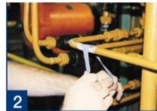
2 remove paint and clean pipe
