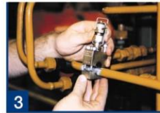
3 clamp SC onto pipe
